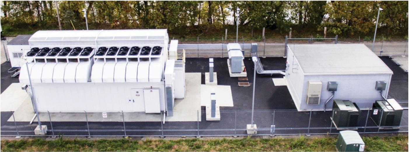
This EcoPOD was assembled on site in three months, providing space for 44 racks that accommodated up to 24,000 hard drives, and featured security, fire suppression, and monitoring systems. It offers energy-efficiencies, such as an adaptive cooling system, to help keep operational costs down.
